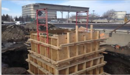
Concrete Forming
